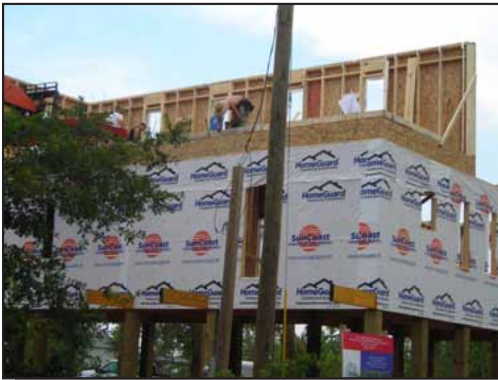
Early construction on two-story model unit.
